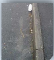
Example of a Grade 'B' Street
